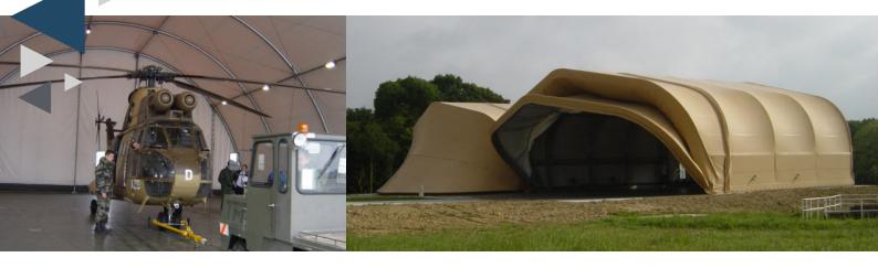
The Hangar System is a large steel structure clad with a PVC cover. These structures are primarily used for aircraft parking and maintenance but can also be used for vehicle garaging or bulk storage. The Hangar is installed permanently or semi-permanently anchored to a flat platform.
